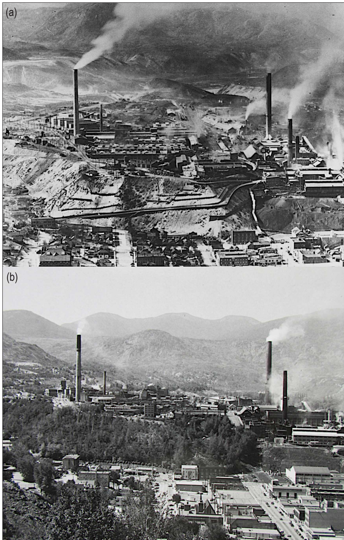
Figure 1. Cominco smelter and area, Trail, B.C., about 1930 (a) and about 1978 (b). The contrast between the bare hillsides in 1930 and the revegetation in 1978 is clear.
